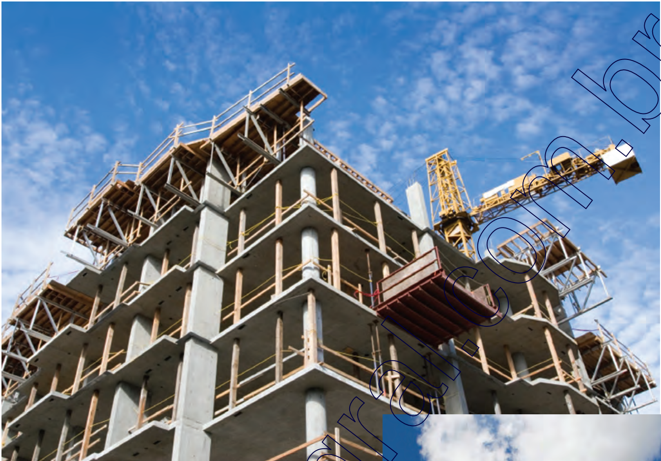
Construction Elevator Emergency Stops
