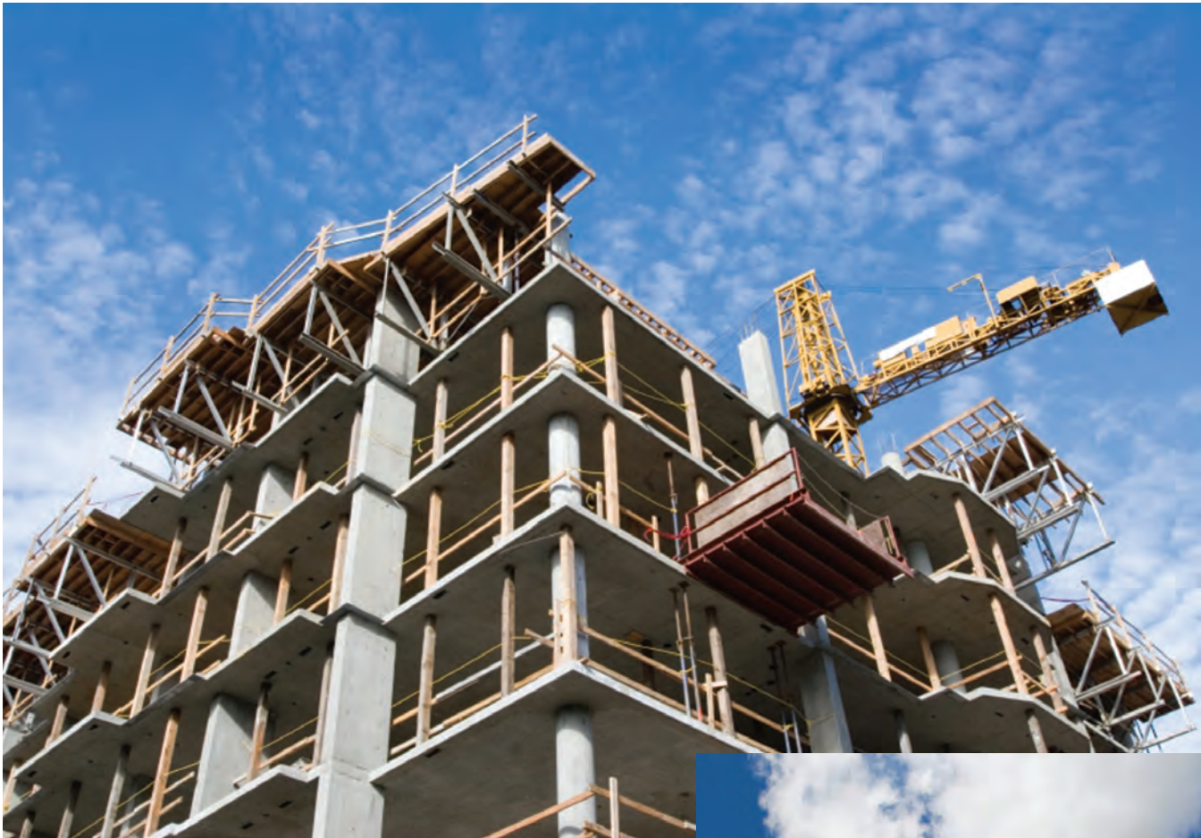
Construction Elevator Emergency Stops
